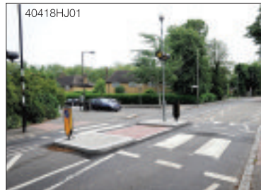
KNOCK-ON EFFECT: The junction of Red Post Hill and Casino Avenue
